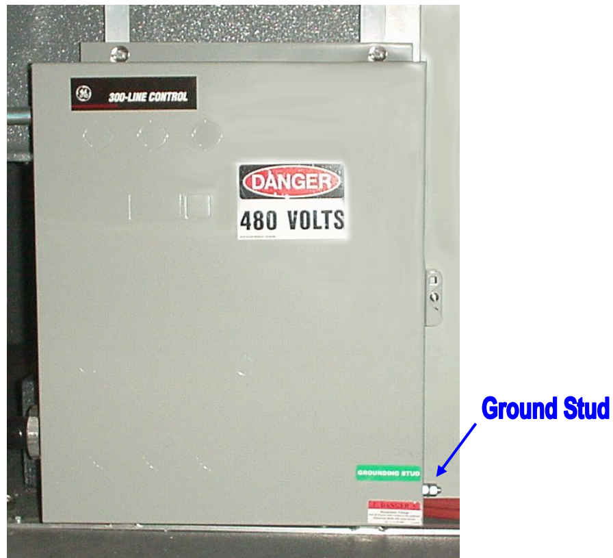
Figure 1: Ground Connection
