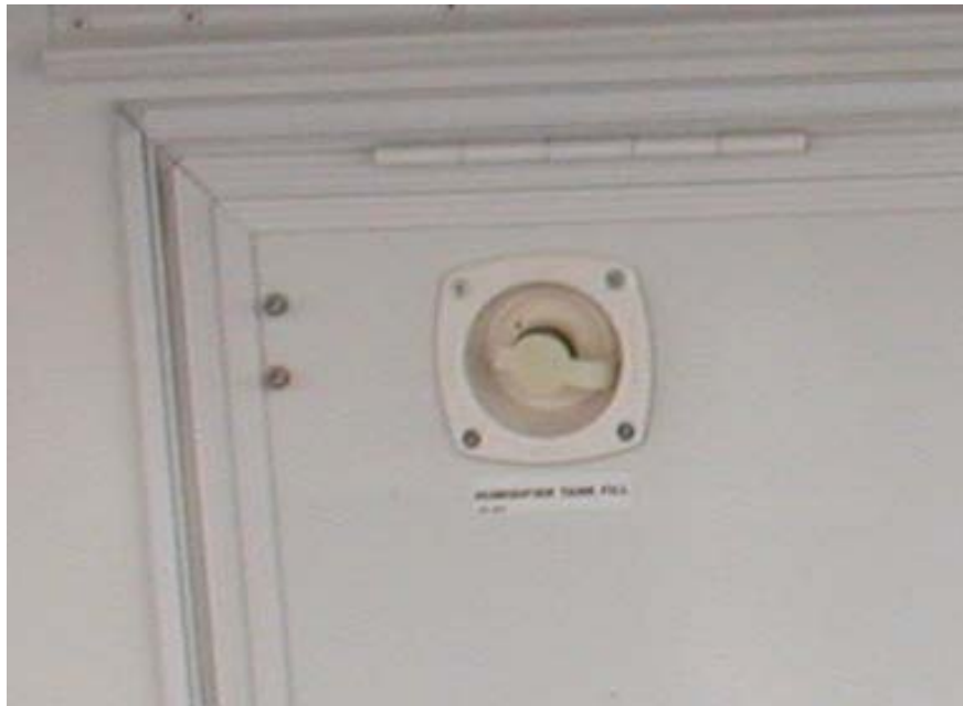
Figure 26: Humidifier Tank Fill
