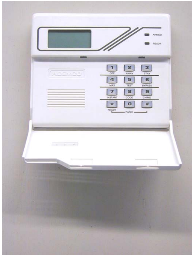
Figure 43: Intrusion Alarm Keypad
