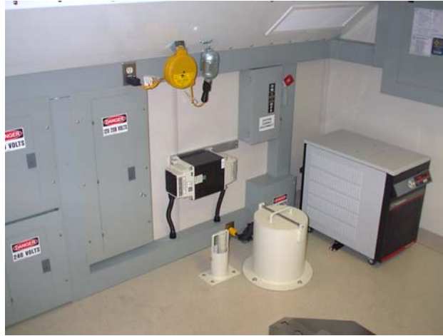
Figure 29: 480V and 120/208V AC Electrical Panels
