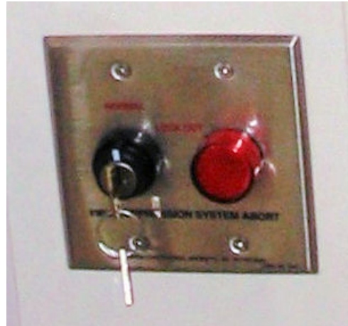
Figure 23: Maintenance Switch
