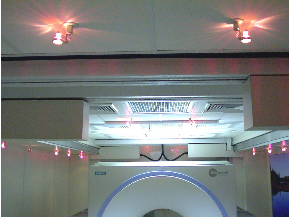
Figure 51: Gantry Room Overall Lighting
