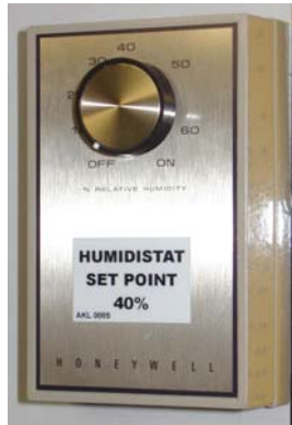
Figure 34: Humidity Controller
