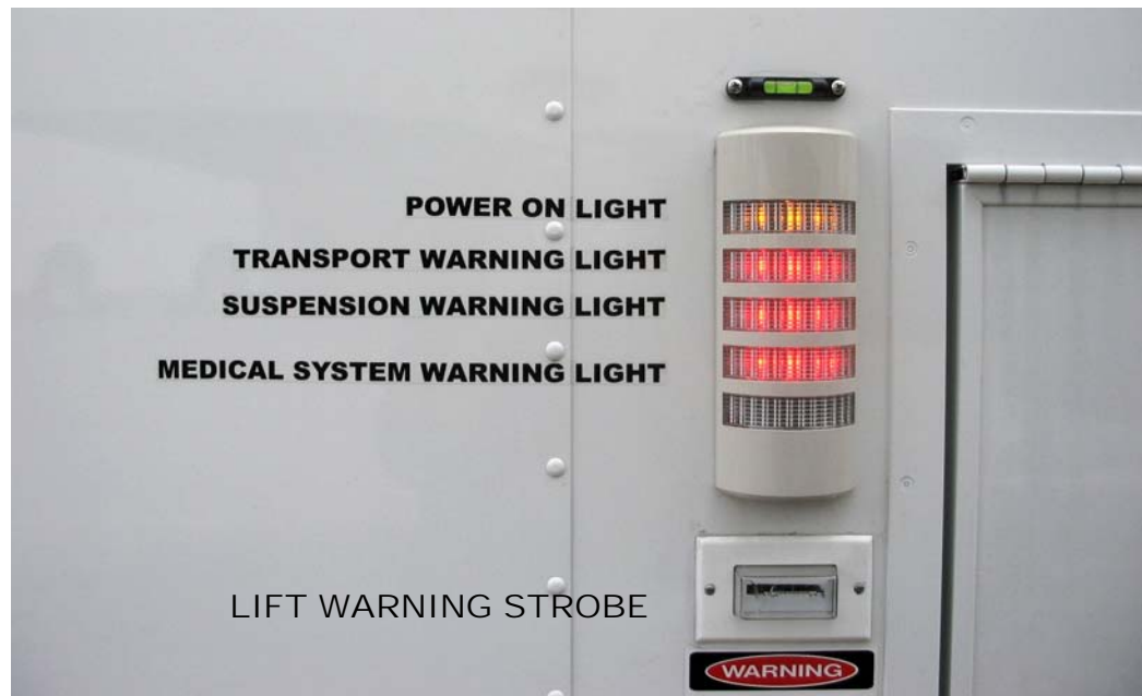
Figure 54: Lift Transport Warning Strobe
