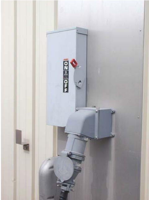
Figure 32: Shore Power Connection
