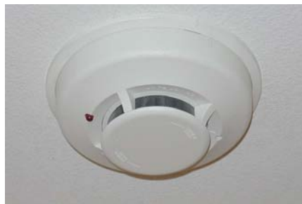
Figure 18: Smoke Detector
