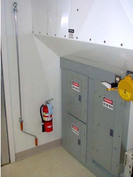
Figure 29: 480V and 120/208V AC Electrical Panels
