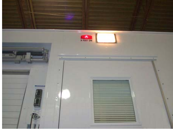
Figure 54: Staff Door Lighting
