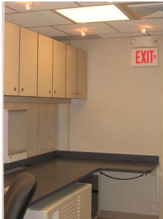
Figure 3: Control Room Overall
